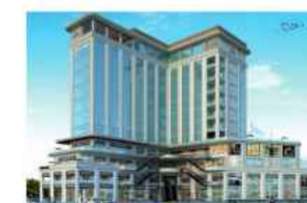
ASHOKA TOWERS SECTOR-63A, GURUGRAM
